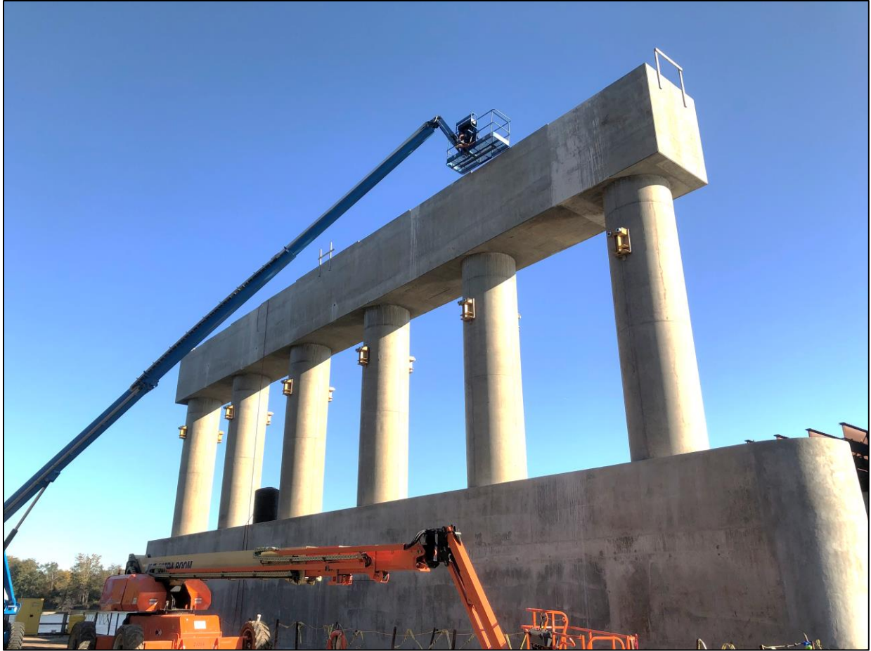
Figure 1: Photo of the tested bridge Pier 1 Pier Cap looking at the west face and visible lift line.
