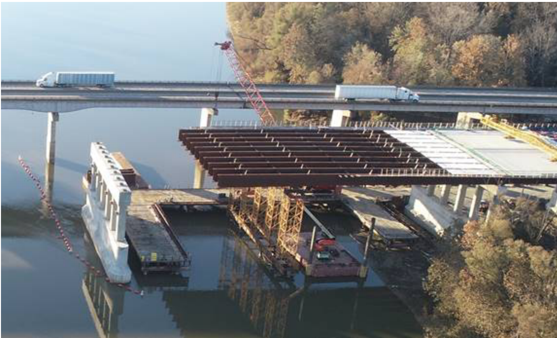
White River Bridge project BB0610 11/2019
