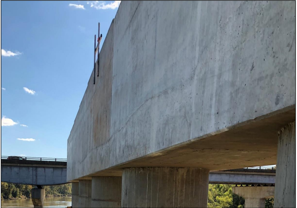
Figure 2: Photo of visible lift line on the East face of Pier Cap 1 looking to south.
