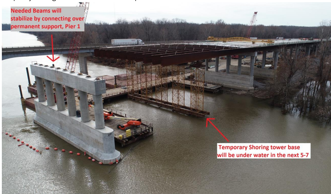
1. Photo of conditions 12/3/19 at White River Bridge jobsite with steel set on temporary shoring towers
