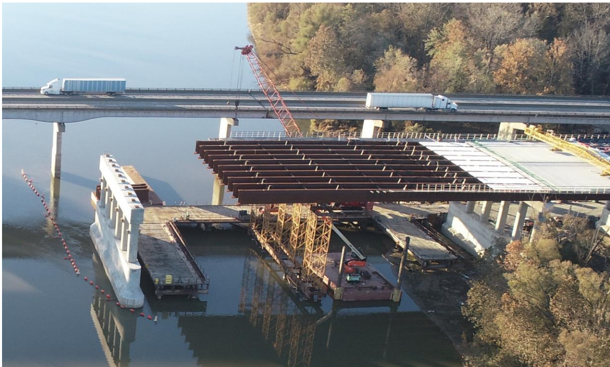
1. Photo of current conditions at White River Bridge jobsite with steel set on temporary shoring towers
