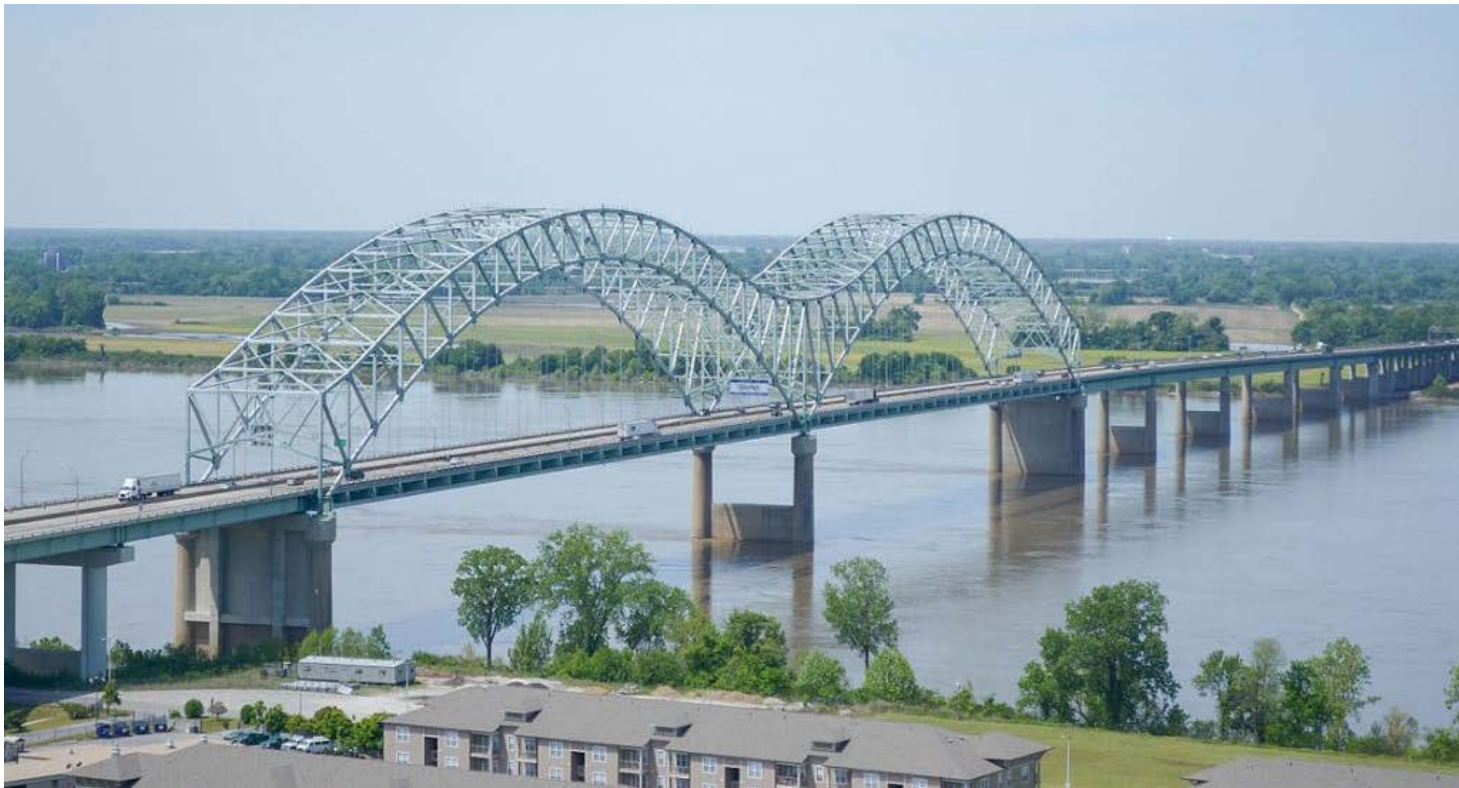
Hernando Desoto Bridge
