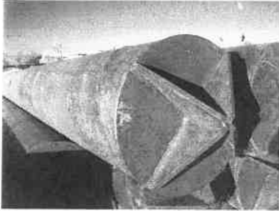
Vaned Tips prior to Driving
