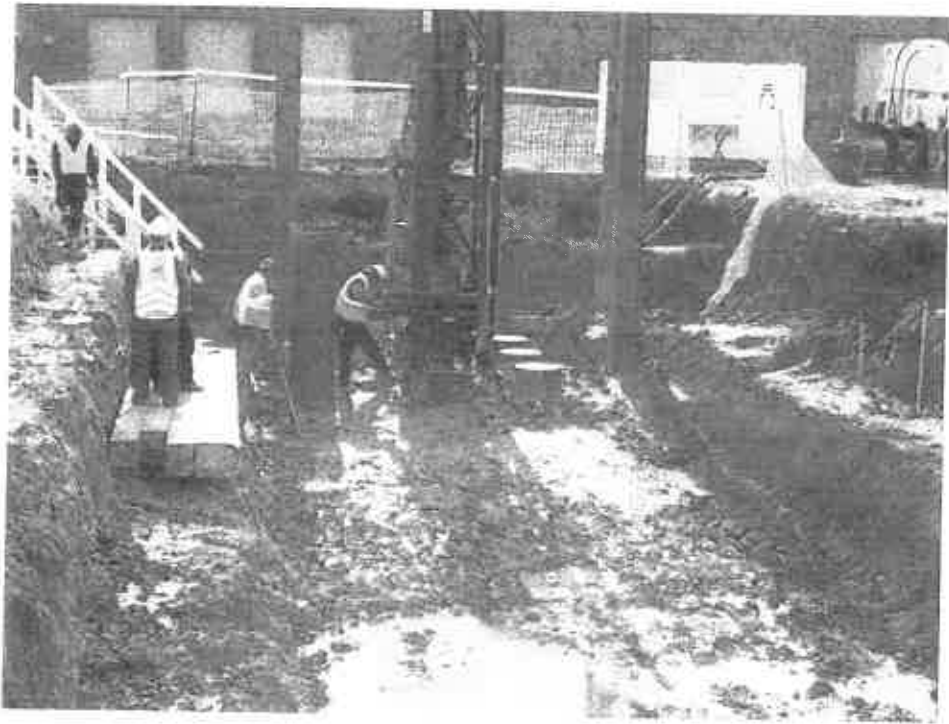
Images of the Delmag Pile Hammer driving pile.
