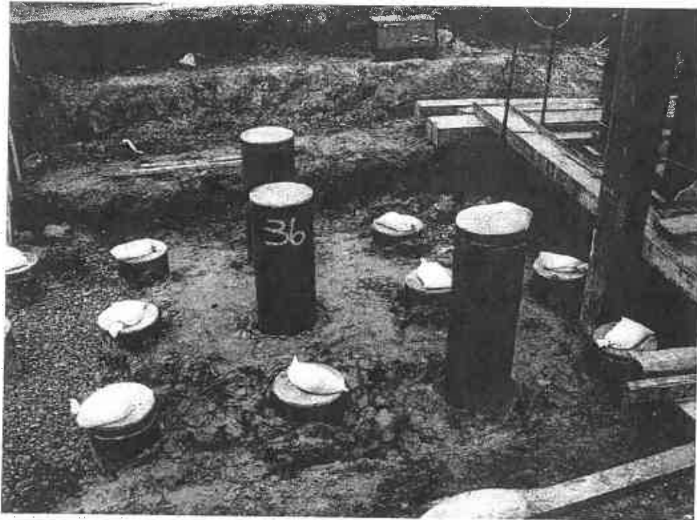
-Concrete-filled steel pipe piling prior to footing concrete placement.
