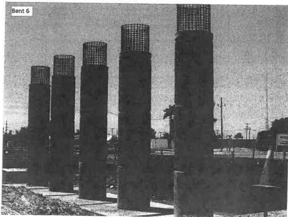
-Reinforced concrete footings and columns.
